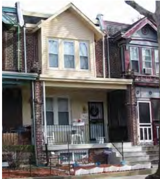
House renovated through the Homeownership Rehabilitation Program
